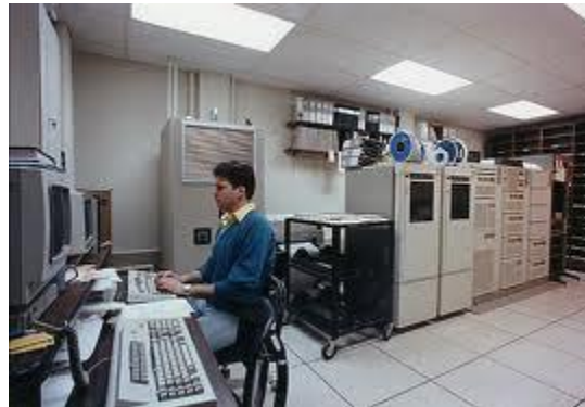
Figure 18: Computer Room Environment
