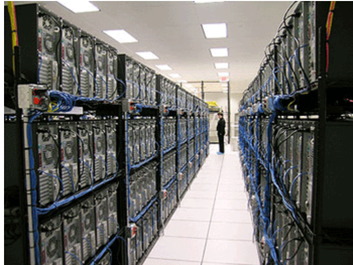
Figure 3: Typical Data Center
